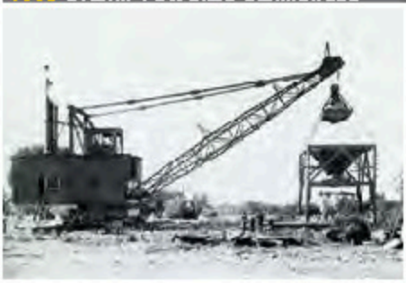
1890 STEAM-POWERED CLAMSHELL
