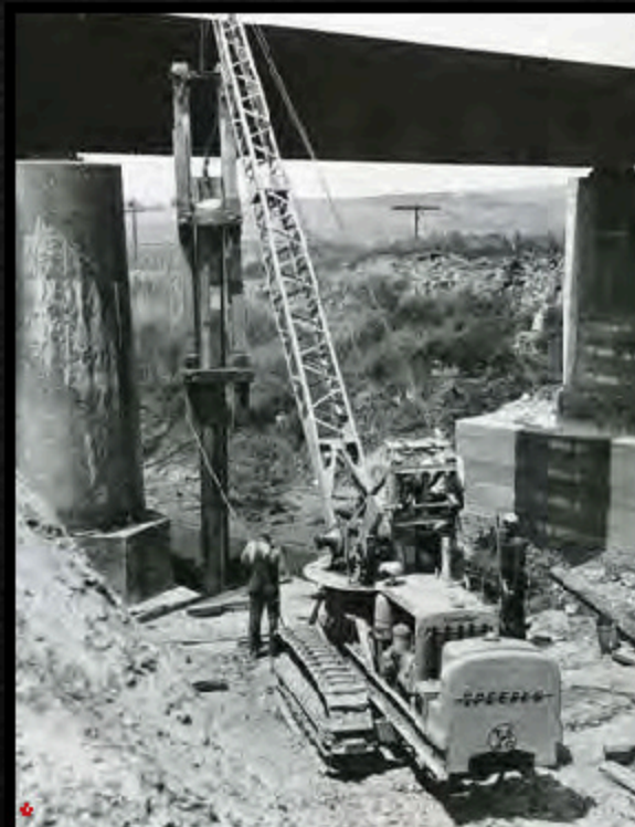
* LINK-BELT SPEEDER TS-40 TRACTOR MOUNTED CRANE DRIVING PILES NEAR RALSTON, NEBRASKA. JULY, 1940.
