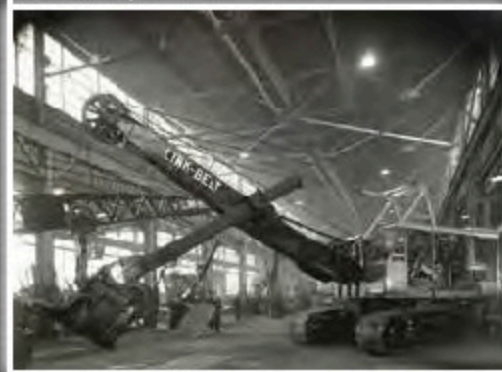
1921 - LINK-BELT BEGAN DEVELOPMENT OF A LINE OF CRAWLER-MOUNTED CRANE-SHOVELS TO COMPLEMENT ITS LINE OF LOCOMOTIVE CRANES AND MATERIAL HANDLING EQUIPMENT.
